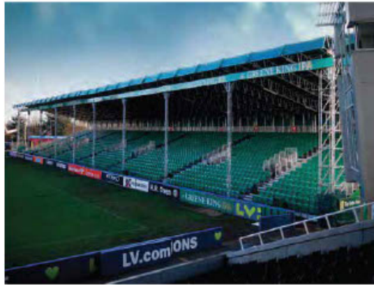
Temporary Scaffold Type Roof
