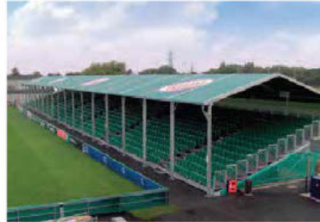
Temporary Marquee Type Roof
